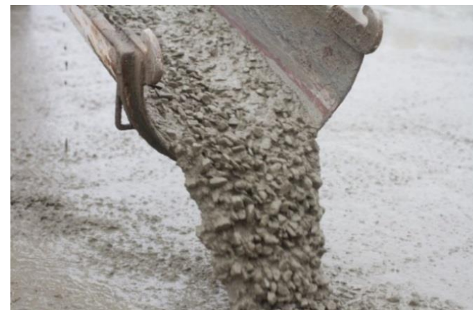
Control Flow Concrete being placed in a flatwork application
