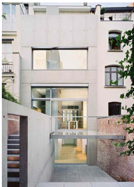
Figure 5e: A cast in situ town house in Brussels, Belgium (Courtesy Architect – Joël Claisse Architectures; Photographer – Jean-Paul Legros, Belgium)
