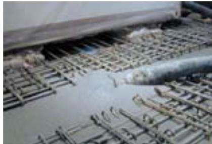
Self-compacting concrete is extremely fluid. It needs no vibration to compact and is easier to place, which is better for workers' health and safety and saves time. Courtesy of BFBN.
