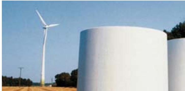
Precast concrete is often used for wind turbines - its high level of weather resistance and inherent stiffness help provide a stable and resilient structure that generates electricity, which is a renewable resource. Courtesy of British Precast
