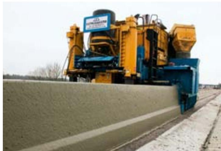
Concrete safety barriers are now being used on all motorways in the UK. They are designed to achieve an essentially maintenance-free serviceable life of not less than 50 years. Courtesy of Britpave.
