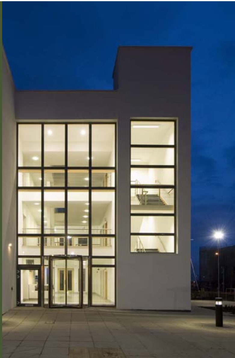
Innovate Office, Leeds utilises the thermal mass of concrete as part of an energy efficiency strategy that has been rewarded with a BREEAM Excellent rating.
